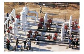
The Custody Transfer Metering system at the delivery point where oil or gas is changing hands forms the basis for invoicing. Every cubic meter of product has to be accurately accounted for, its delivery conditions (such as pressure, temperature, contaminants and energy value) closely monitored and recorded.
